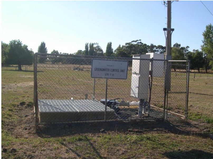
Figure 8: Example of a public groundwater pump
