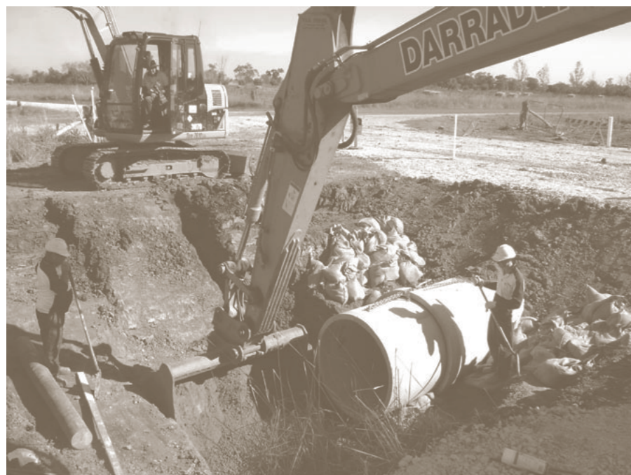
Road culvert replacement on the corner of Mason Rd and Morrissey Road, Stanhope.
