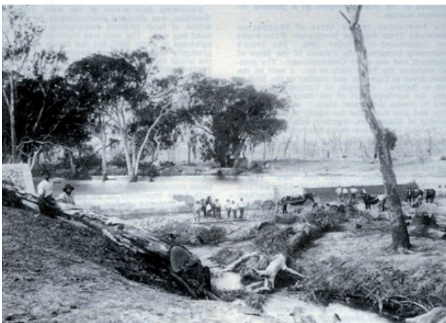
Construction of the Gowangardie Weir. circa 1897 from "Shepparton Shire Reflections".
