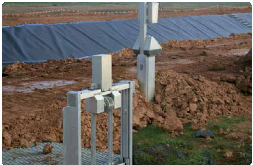
Channel remediation works with a 450mm Magflow Meter with automated SlipGate
