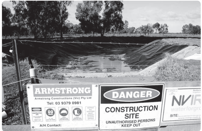
Plastic Lining Murray Valley no. 7/2 channel, Mywee
