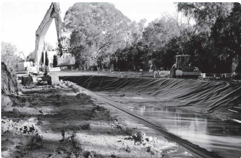
Plastic Lining Murray Valley no. 7/2 channel, Mywee
