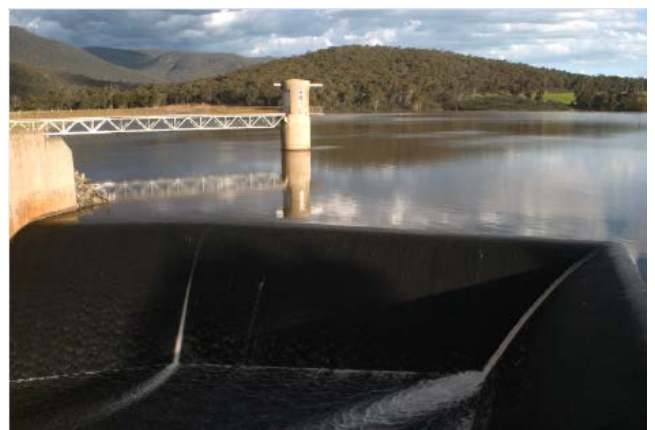
Lake Nillahcootie outlet tower and spillway
