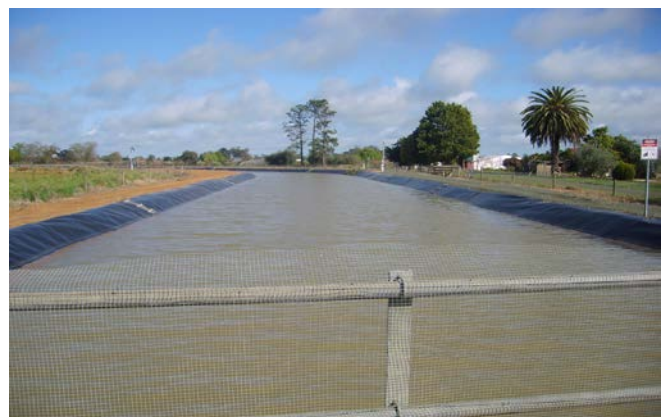
Plastic lined channel at Tongala
