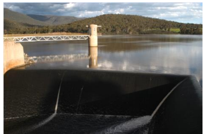
Lake Nillahcootie outlet tower and spillway
