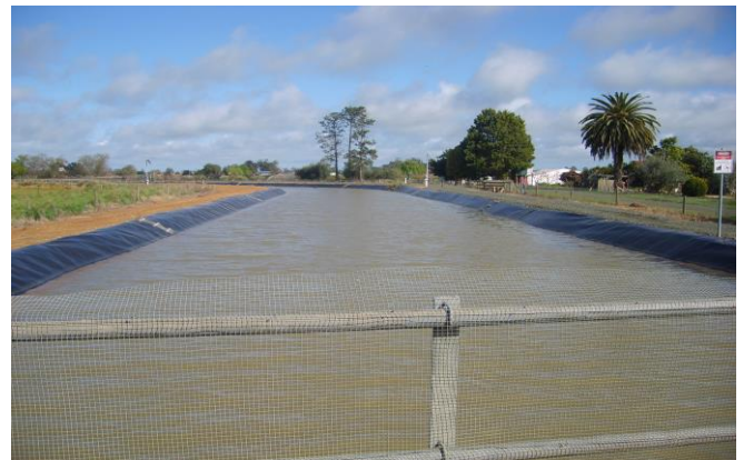
Plastic lined channel at Tongala
