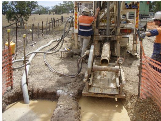
Drilling of a State monitoring bore
