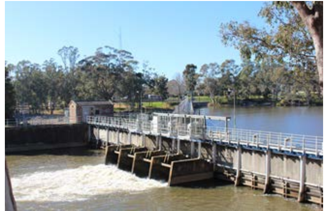
The Stuart Murray Canal offtake and the Goulburn Weir.
