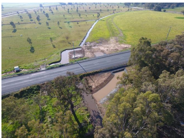
Photo 1: Upper Deakin catchment – completed works now connect drainage flow paths under Midland Hwy, Stanhope
