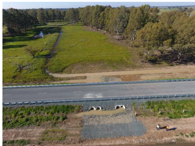
Photo 2: Upper Deakin catchment – works at McEwen Rd, Stanhope have removed obstructions to natural drainage
