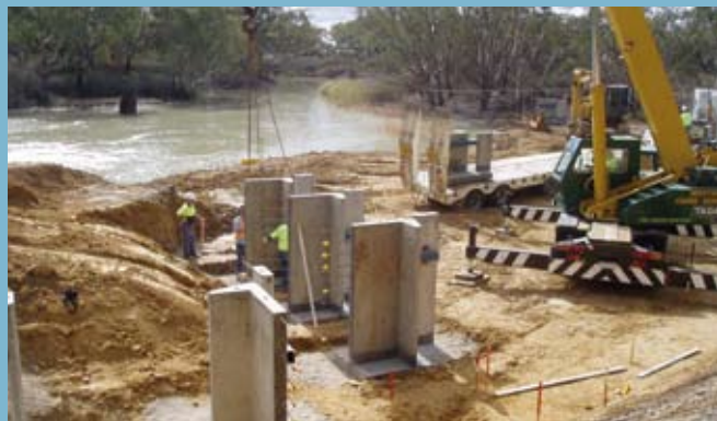
Kerang Weir Fishway Funded by North Central CMA. Construction of the concrete fishway structure alongside the Kerang Weir on the Loddon River commenced in April 2008.
