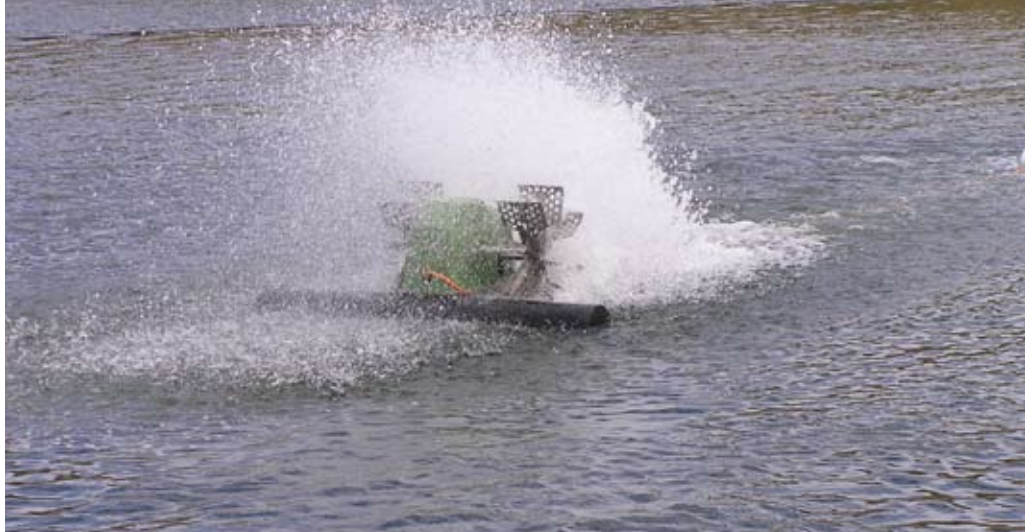
G-MW installed and ran aerators at Lake Eppalock and Lake Tullaroop to combat water quality issues created by record low storage levels.
