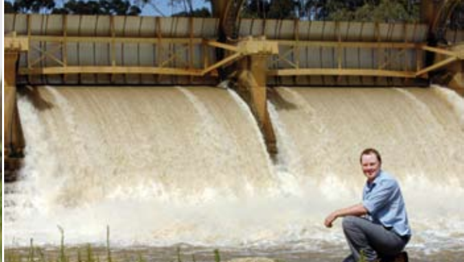
G-MW's Senior Reservoir Officer Goulburn Weir, Michael Wilkman, at Goulburn Weir.
