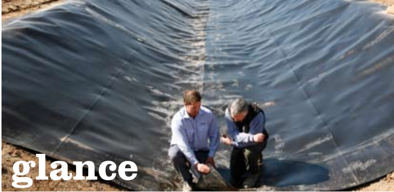
G-MW's FutureFlow began lining 28 km of channel as part of its 2008 works program.
