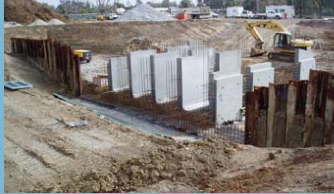
Gunbower Weir Replacement and Fishway; G-MW commenced works to replace the Gunbower Weir, north-west of Echuca, in the Torrumbarray Irrigation Area. The Weir was built in the 1890s and has a key role in regulating flows from the National Channel into the Gunbower Creek which supplies irrigation water to Cohuna. A fishway is to be constructed once the weir replacement is complete.
