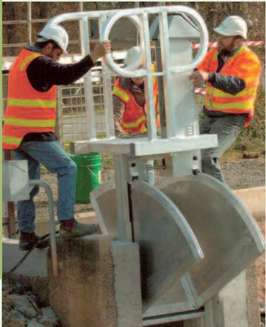
Installing channel automation technology in the Central Goulburn area
