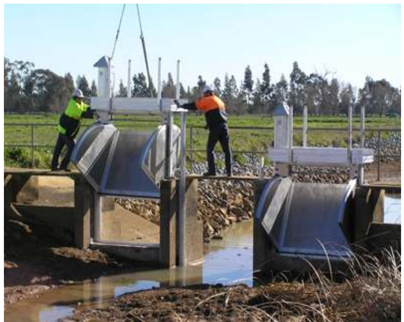
Installing automated regulators in the Shepparton Irrigation Area
