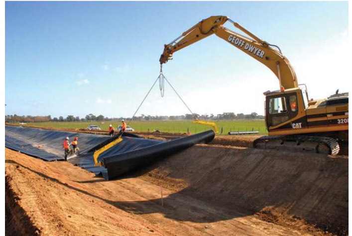
Installing HDPE channel lining during 2008 Winter works program
