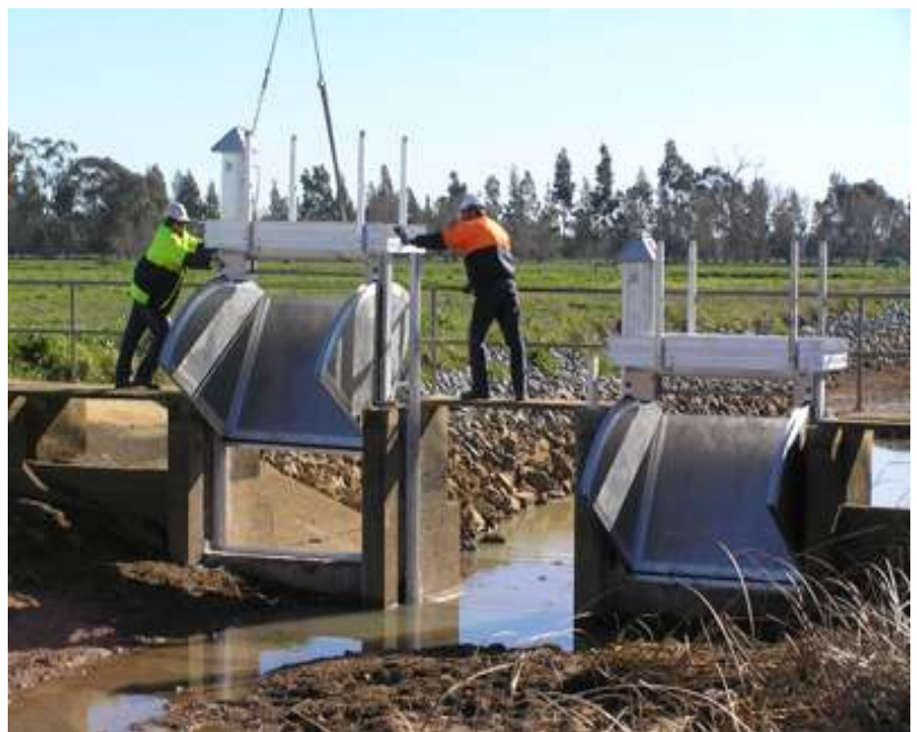
Installing automated regulators in the Shepparton Irrigation Area
