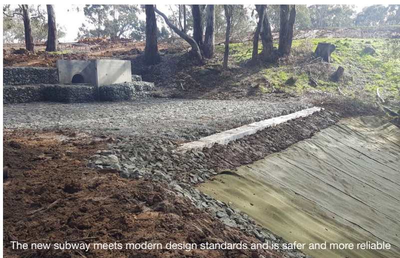
The upgrade replaced the aging subway
