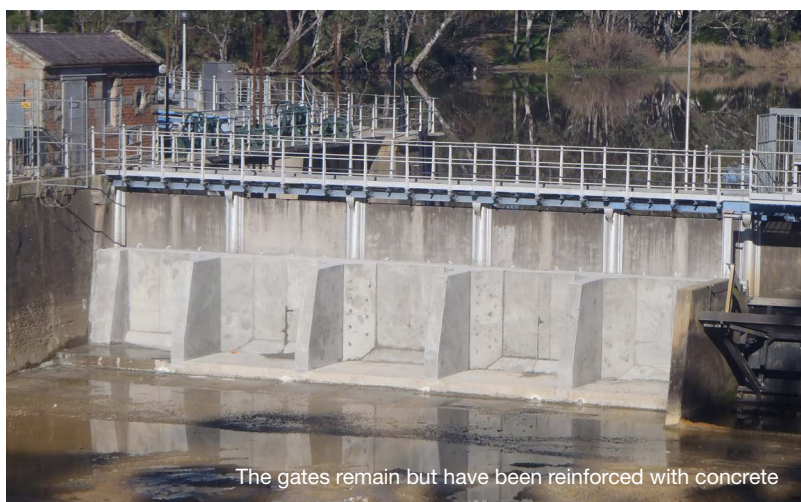
The offtake structure was stabilised and the vertical drive gates were decommissioned
