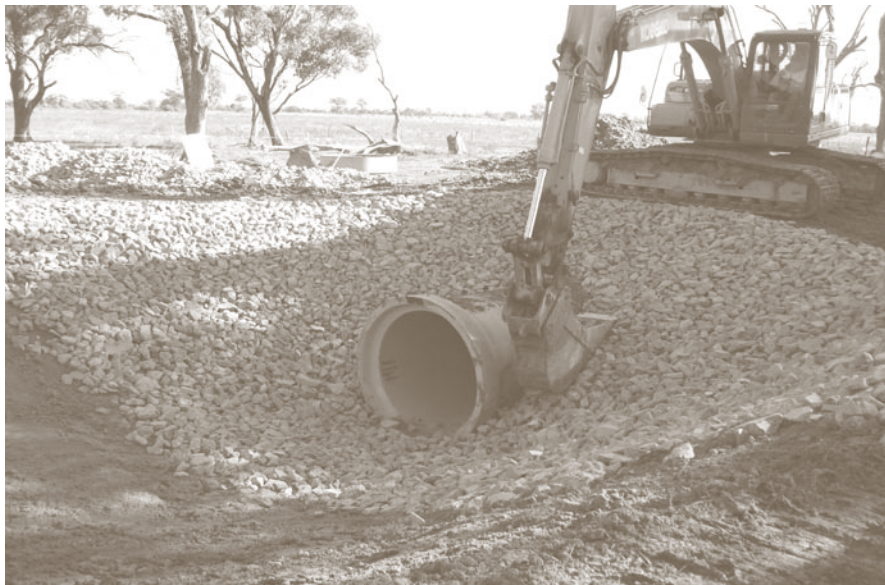
Replacing an occupation crossing on channel 17.
