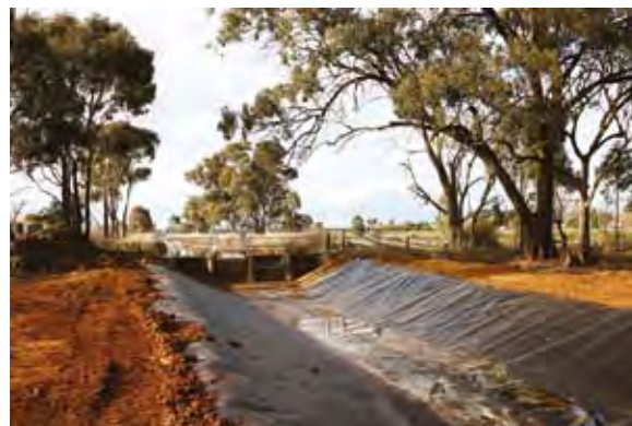
Commencement of Central Goulburn channel lining
