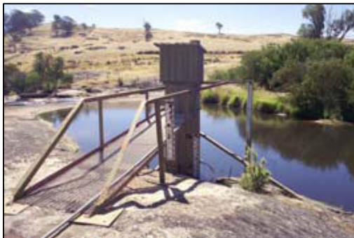
Figure 10- Gauging station at Polly McQuinns weir (Thiess)
