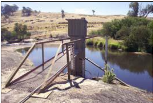
Figure 10- Gauging station at Polly McQuinns weir (Thiess)
