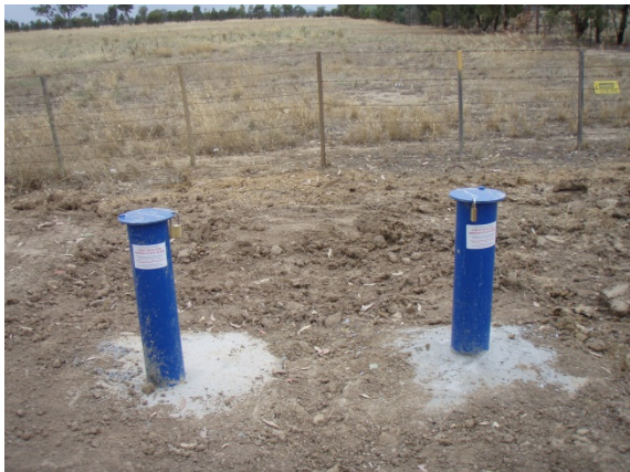
Nested State monitoring bores at Murchison
