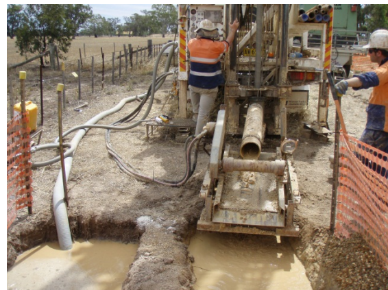
Drilling of a State monitoring bore
