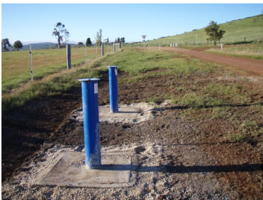
Nestled State monitoring bores at Lauriston
