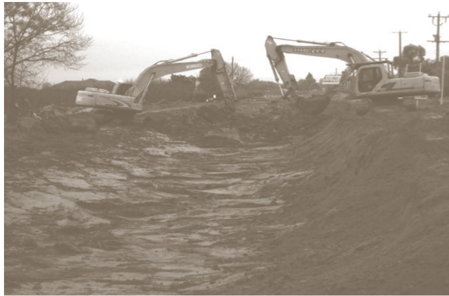
Contractors preparing the MV No 1 channel for plastic lining near Cobram.
