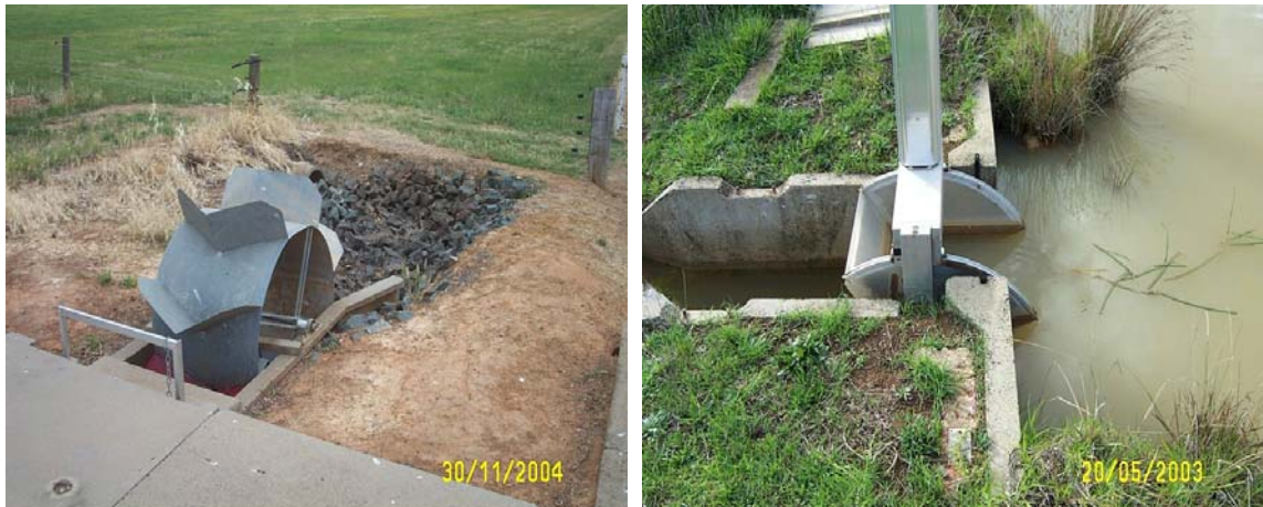
Figure 3 - Comparison of Dethridge Wheel and FlumeGate™
