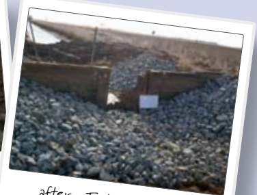
after... Typical Structural Rehabilitation
